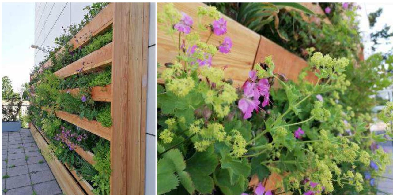
Fig. 3 and 4: EVAPO+ transpiring green wall on the roof terrace of the Strasshof municipal office
