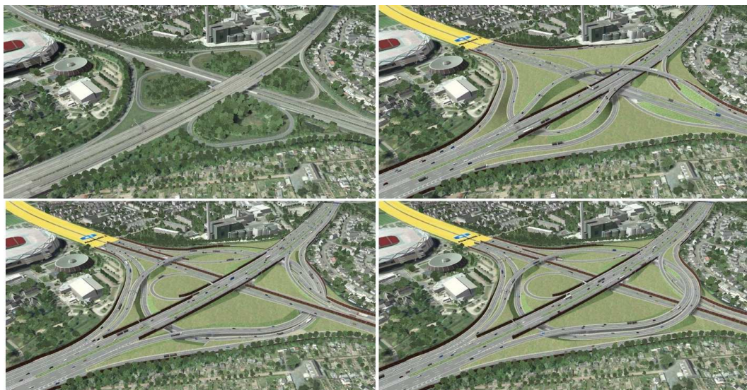
Figure 5: Variant analysis for an interchange. Only the relevant geometry and animation is exchanged.
