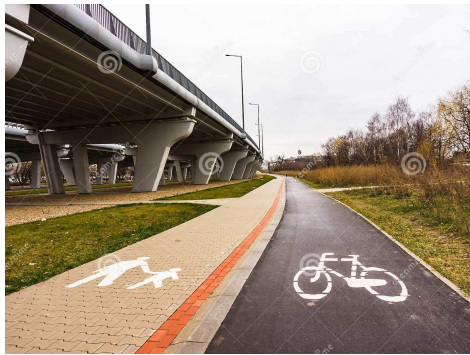
Fig. 1: An Image of a Bike Route and Footpath with Symbols Along a Bridge at a Park in Poznan, Poland (Source: Dreamstime, 2019)
