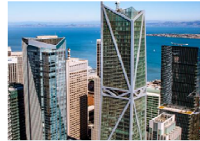
181 Fremont Street San Francisco, USA
