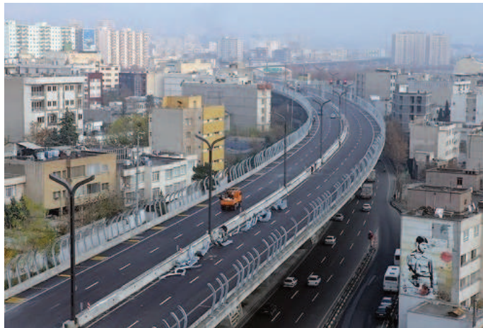
Fig. 7: Sadr Elevated Highway
