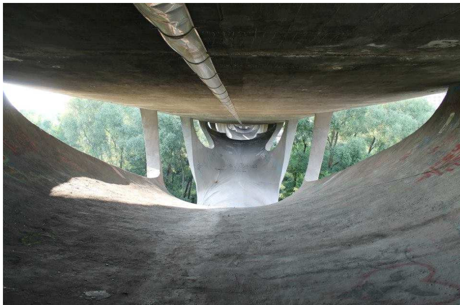
Fig. 2: The underside of Musmeci Bridge.
