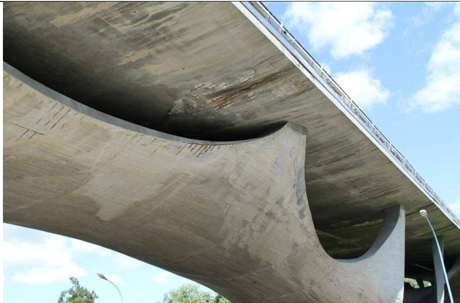
Fig. 5: An external view of Musmeci Bridge.
