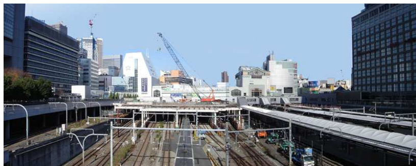
Fig. 3 South Terrace, Shinjuku station, Tokyo
