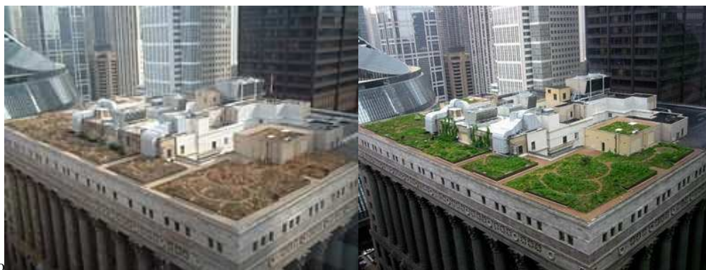
Fig.1. Green roof of Chicago City Hall, Illinois – in early spring and late summer
